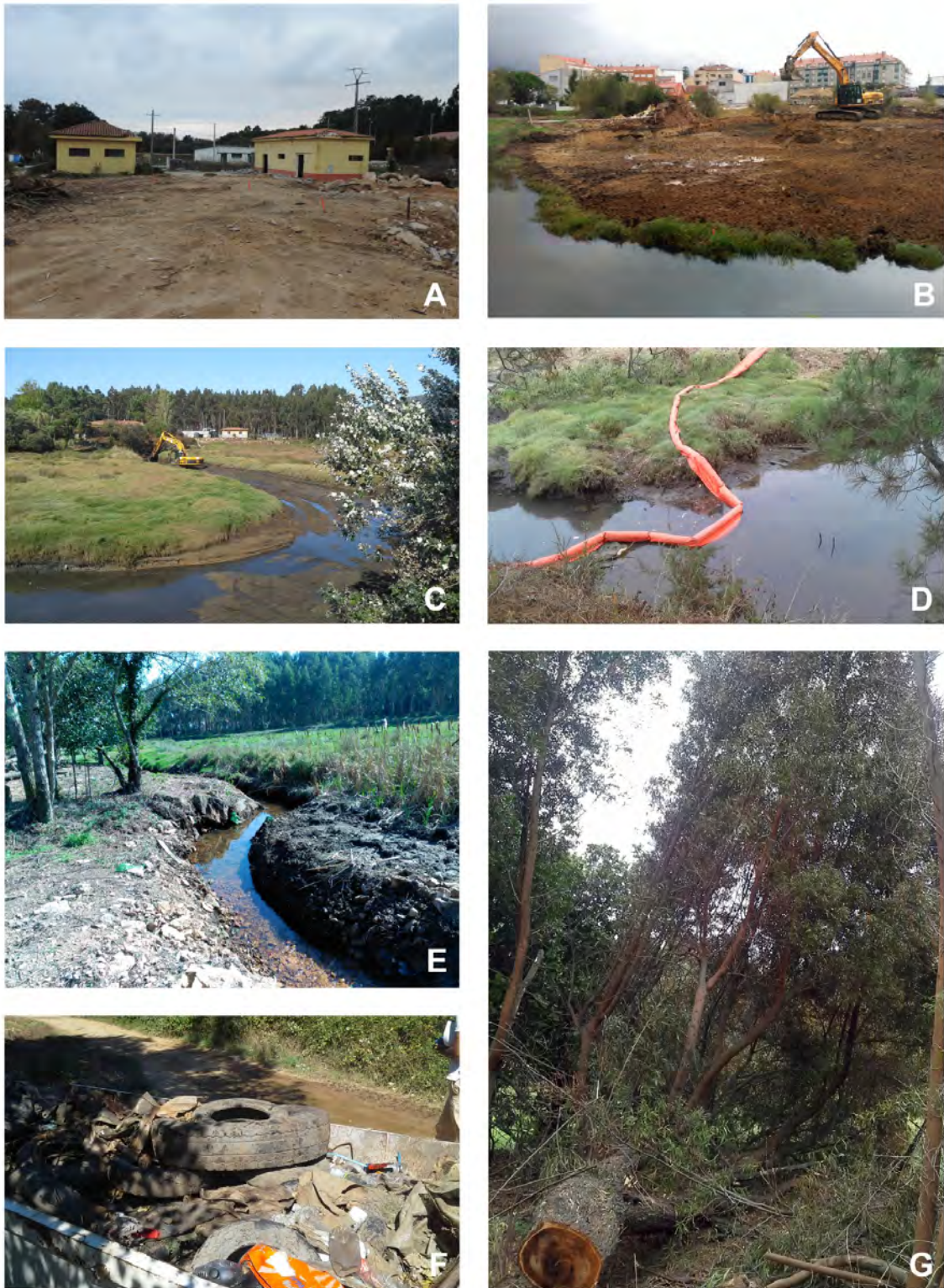
Figure 2. Summary of activities carried out for the restoration of the environmental quality of the Pobra do Caramiñal saltmarsh. A) Overview of the old wastewater treatment plant built in the saltmarsh (filled area 3; Figure 1). This plant was removed and part of the saltmarsh was restored (Figure 1 B); B) Removal of filled area 2 (Figure 1); C) Dredging of polluted sediment; D) Protection barriers for containing suspended materials during sediment dredging; E) Hydrological restoration. Recovery of secondary channels within the saltmarsh; F) Removal of urban solid waste; G) Removal of invasive plant species and restoration of the riparian forest.
